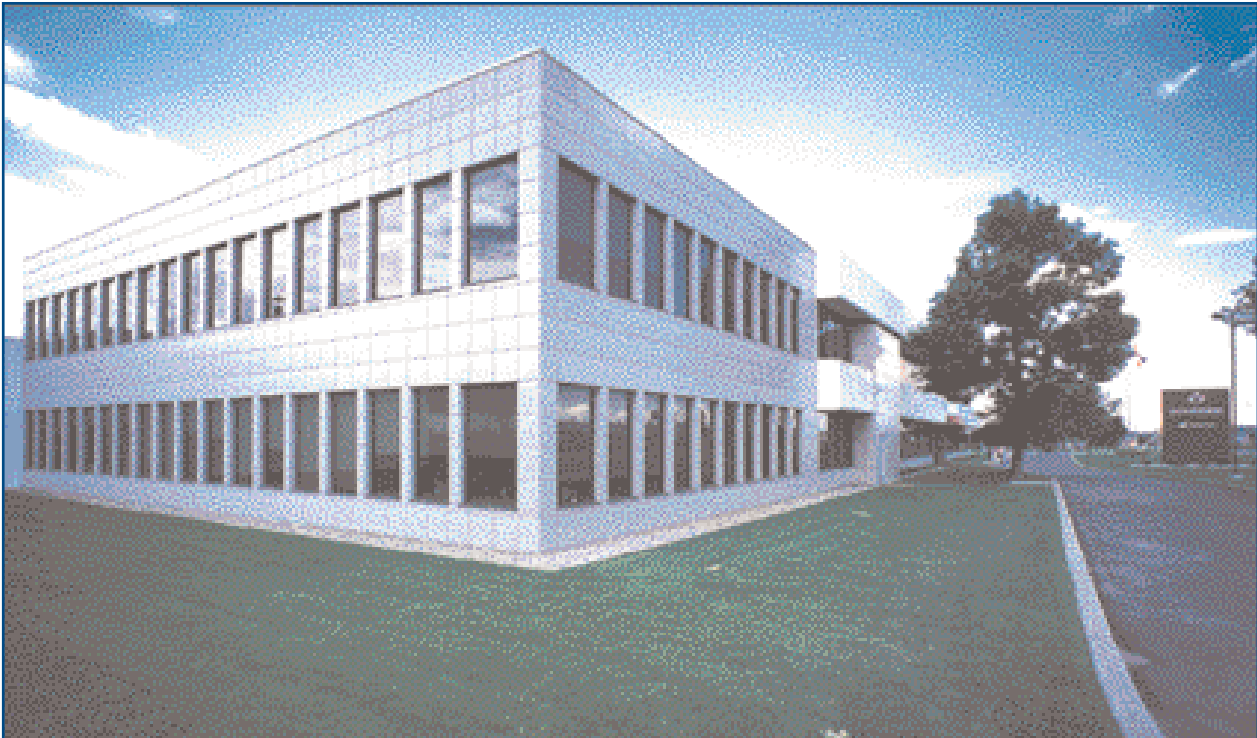
Schering Canada's recently expanded head office and manufacturing plant, Pointe-Claire, Quebec.
